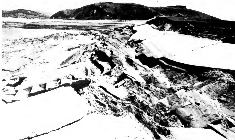
Photo 2. Slide damage at east end of embankment, Lower San Fernando Dam.
